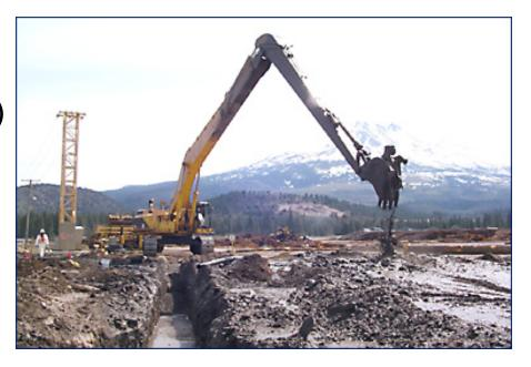
Remedy included TI waiver, slurry wall, pump-and-treat system for containment, long-term monitoring, and institutional controls
