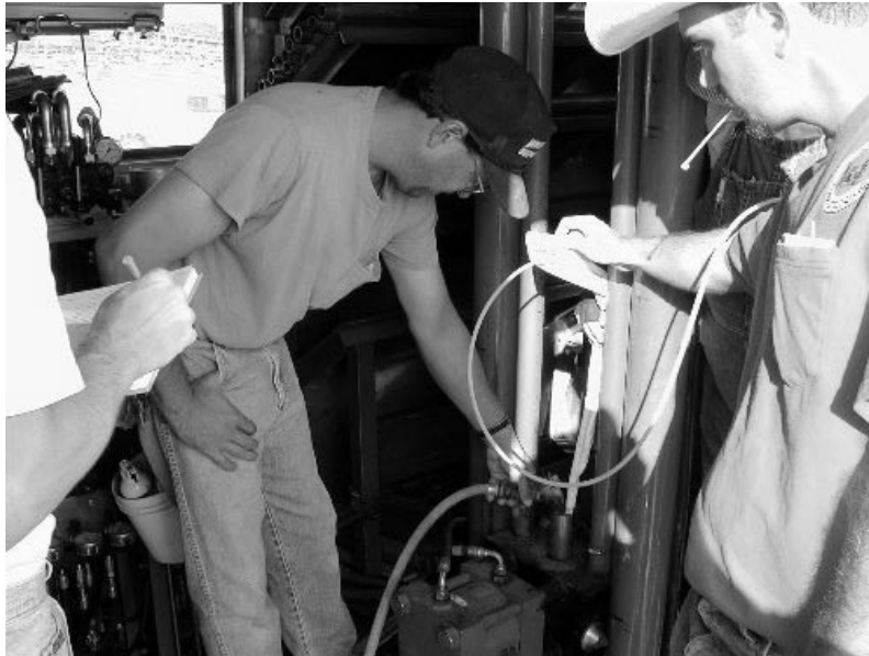
Figure 4. Water is added to the membrane system.
