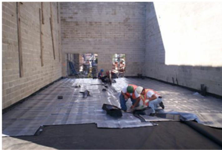
Figure 14-4. Passive Vapor Barrier Installation (Source: DON, 2010)
