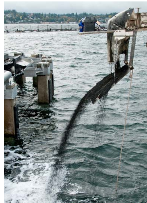
Distributing in berthing area
