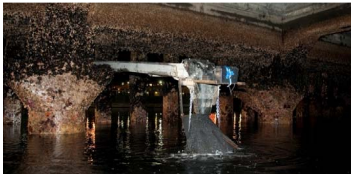
Distributing under pier
