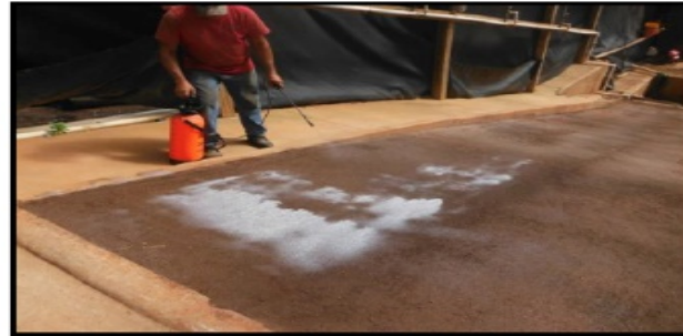
Mixture Sprayed at 1 gallon / 10 sf
