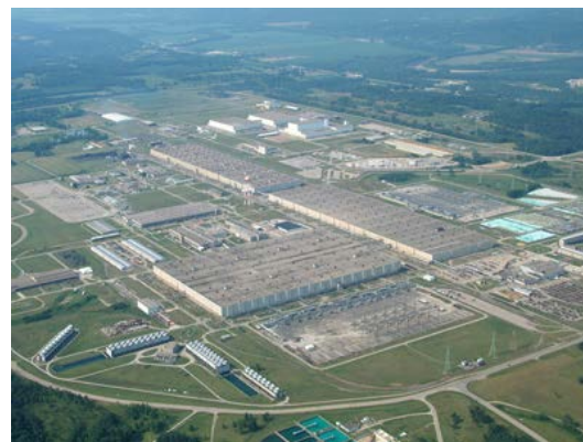
Portsmouth Gaseous Diffusion Plant
