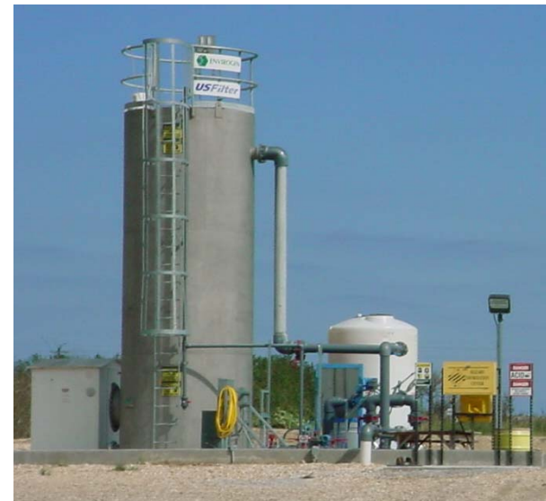
Fluidized Bed Reactor
