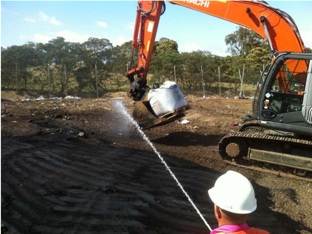
Laying the Amendment Capping Layer
