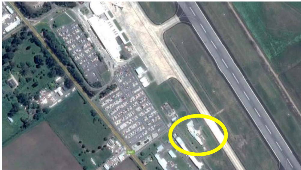
Aviation Rescue and Fire Fighting Services
