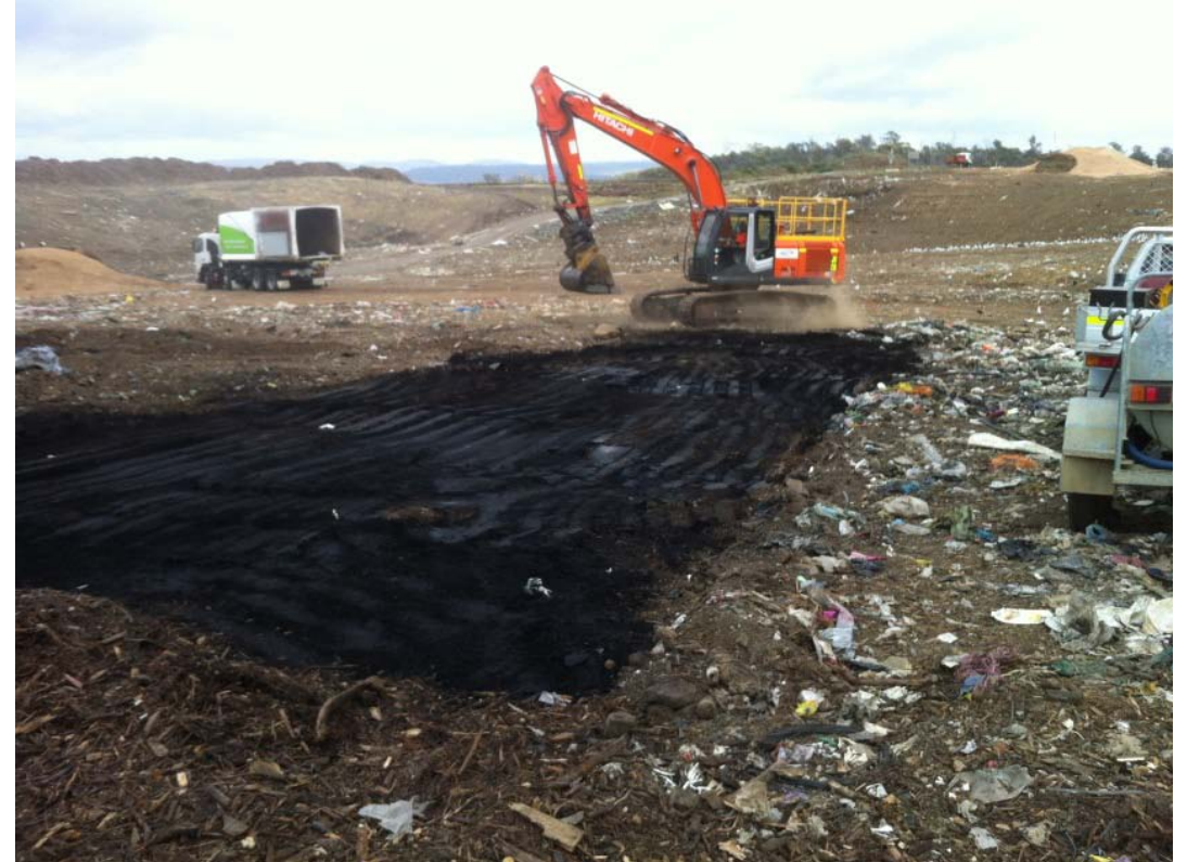
Finished Lined Burial Cell
