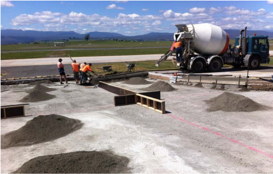
Construction of New Apron
