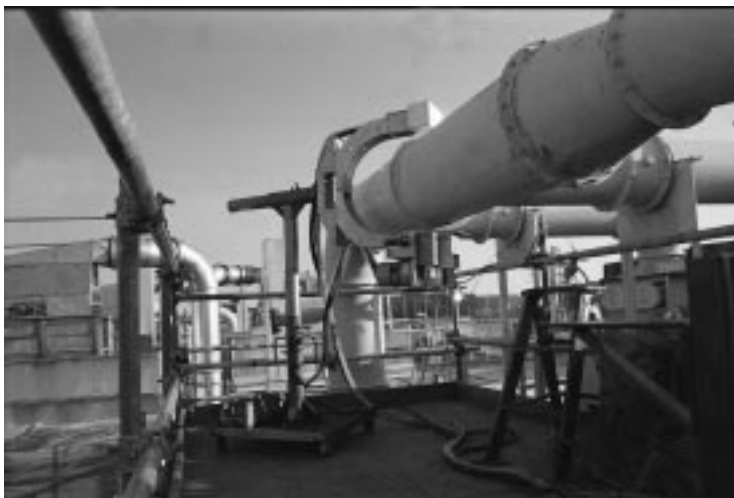
Figure 1. Inspection Head on 20-Inch Diameter Ventilation Duct
