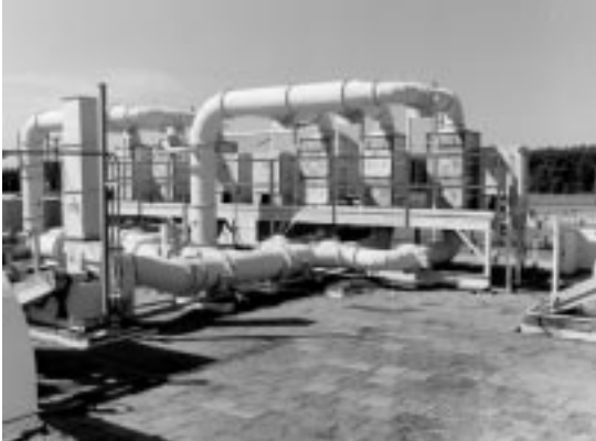
Figure 3. Exhaust System without Scaffolding
