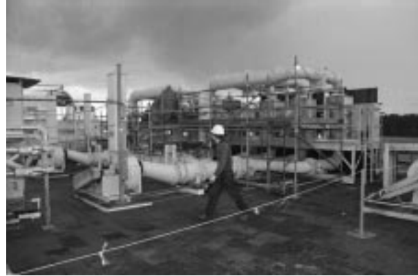
Figure 4. Exhaust System with Scaffolding
