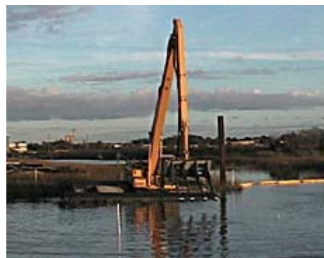
Figure 3. Marsh excavator mixing grout into sediment [1]
