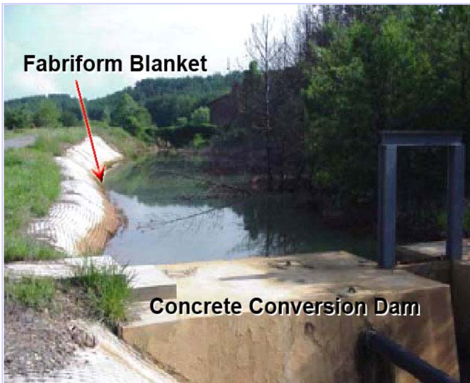
Figure 5: Fabriform Blanket and Conversion Dam
