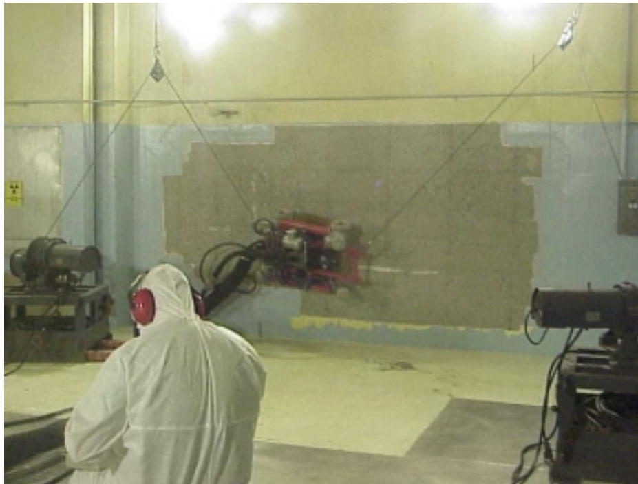
Figure 5. En-vac removing paint from wall in the Decon Shop
