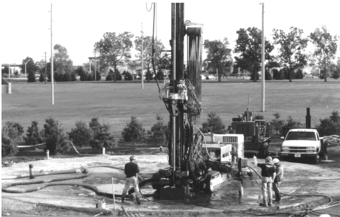
Figure 3. Photograph of jetting rig at the demonstration site.
