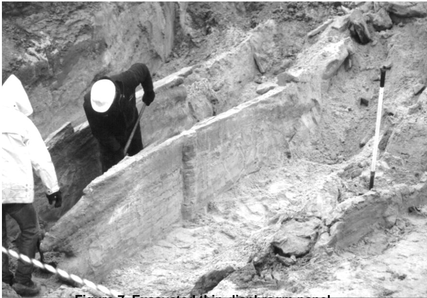
Figure 7. Excavated thin-diaphragm panel emplaced using high-pressure jet grouting.
