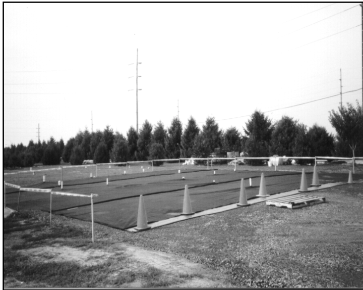
Figure 6. Photograph of the geomembrane cover and piezometers.
