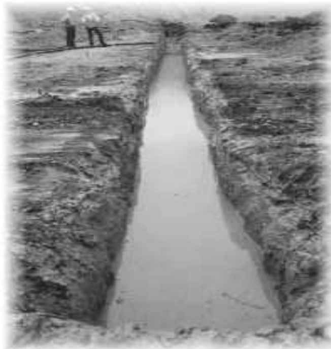
Figure 8. Impermeable wall construction.
