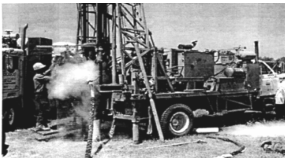
Figure 3. Cryogenic Drilling in Operation
