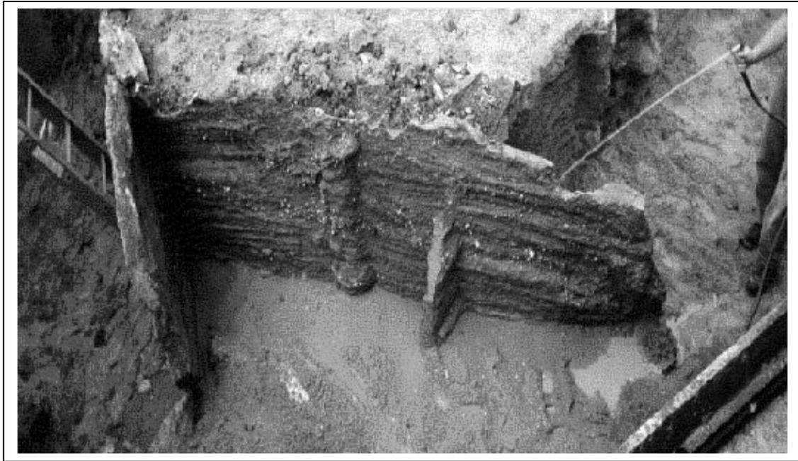
**Figure 6. After examining three-dimensional ERT images at the Dover test site, a portion of a contaminant migration barrier was excavated for further evaluation. Electrical resistivity changes were imaged as salt water tracer moved through the barrier at locations later found to be defects in a wall or the joining of two walls.**
