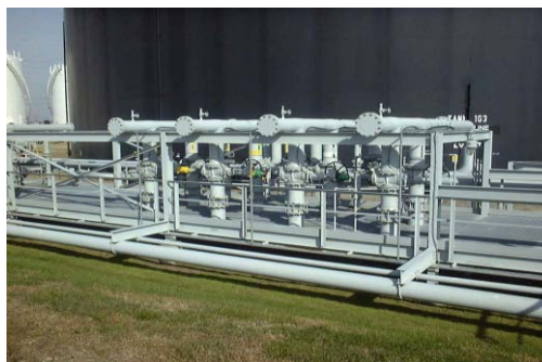
Distribution Piping and Manifold
