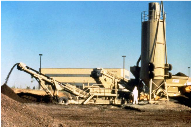
Figure A-3. Pugmill mixing S/S treatment for lead-contaminated soil at 90 th South Battery Site, West Jordan, Utah. Source: S3 Engineers LLC.
