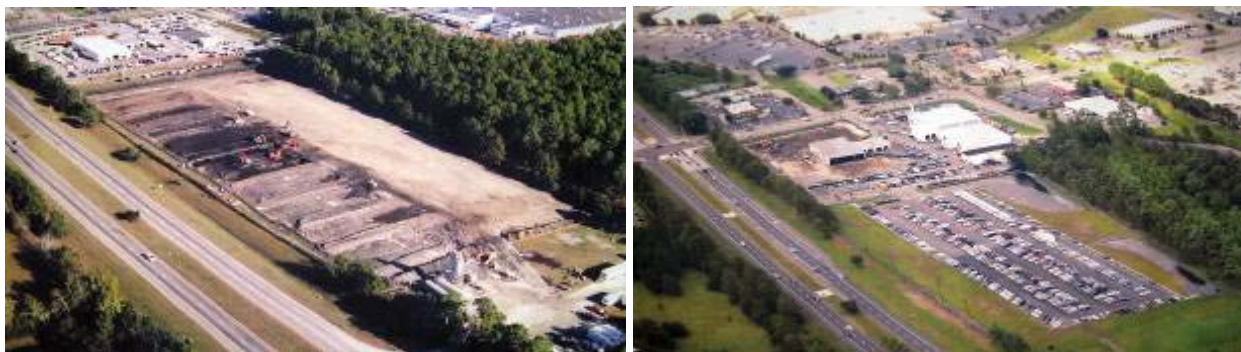
Figure 8-3. Hercules 009 Landfill Superfund Site near Brunswick, Georgia, during S/S treatment (left) and redeveloped into an automobile dealer parking lot. Source: Portland Cement Association, Lear and Wilk 2008.
