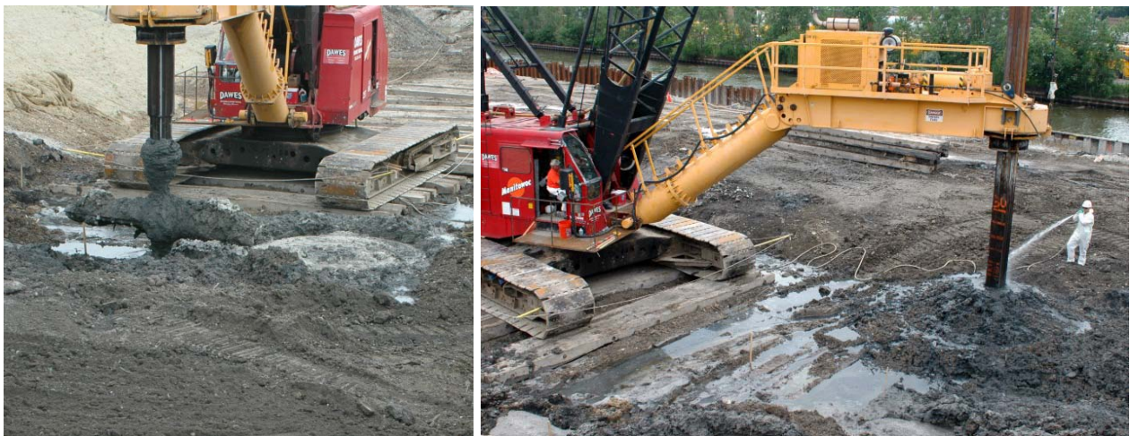
Figure A-11. S/S treatment using an auger with mixing blades exposed (left) and at a depth of 22 feet as indicated by markings on auger shaft, at a former MGP plant, Milwaukee, Wisconsin. Source: Portland Cement Association.
