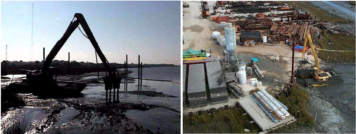
Figure A-9. Rake injector (left) and grout plant and rake injector (right) for treating contaminated sediment at Koppers Co., Inc. (Charleston Plant) Superfund Site, Charleston, S.C. Source: Williams Environmental Services, Inc.
