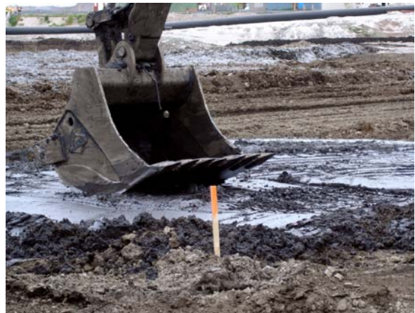
Figure A-8. Finished surface after excavator bucket mixing, Sydney Tar Ponds, Nova Scotia. Source: CETCO Contracting Services Co.
