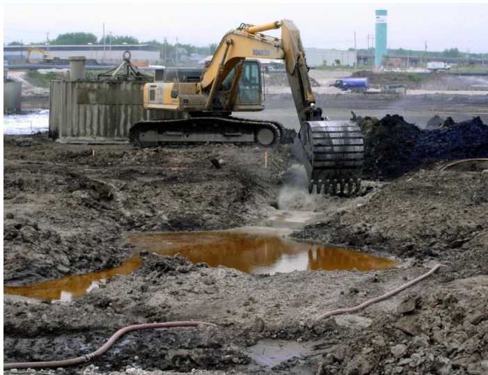
Figure A-7. Excavator bucket mixing of contaminated sediment, Sydney Tar Ponds, Nova Scotia. Source: CETCO Contracting Services Co.
