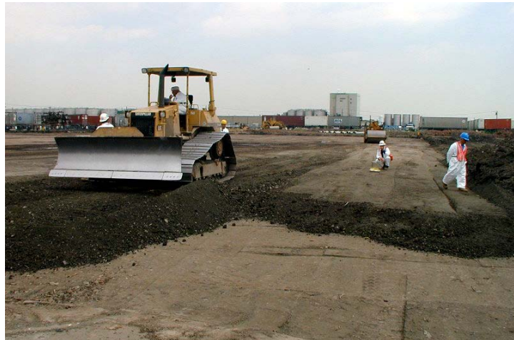
Figure A-2. Pugmilled S/S-treated soil from former wood-preserving site Port Newark, N.J., reused on site as pavement base. Source: Key Environmental, Inc.
