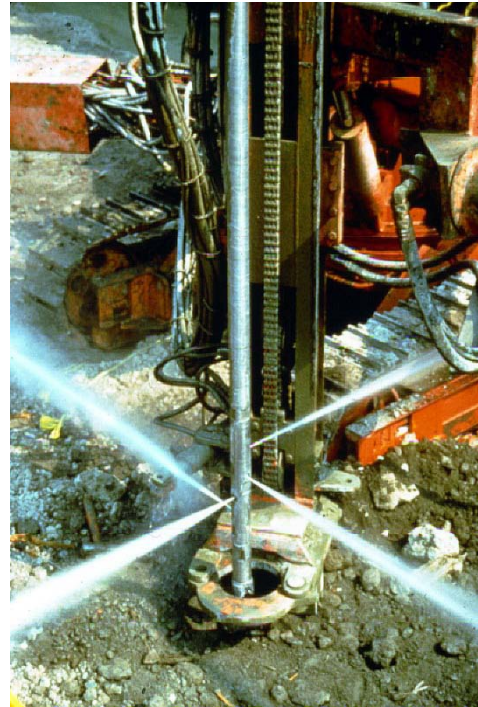
Figure A-12. Jet grouting showing exposed nozzles. Source: Geo-Con, Inc.
