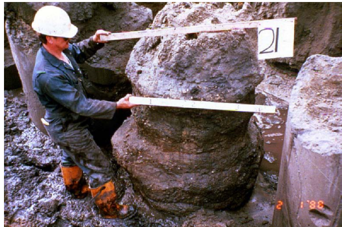
Figure A-13. Exposed jet-grouted columns.
