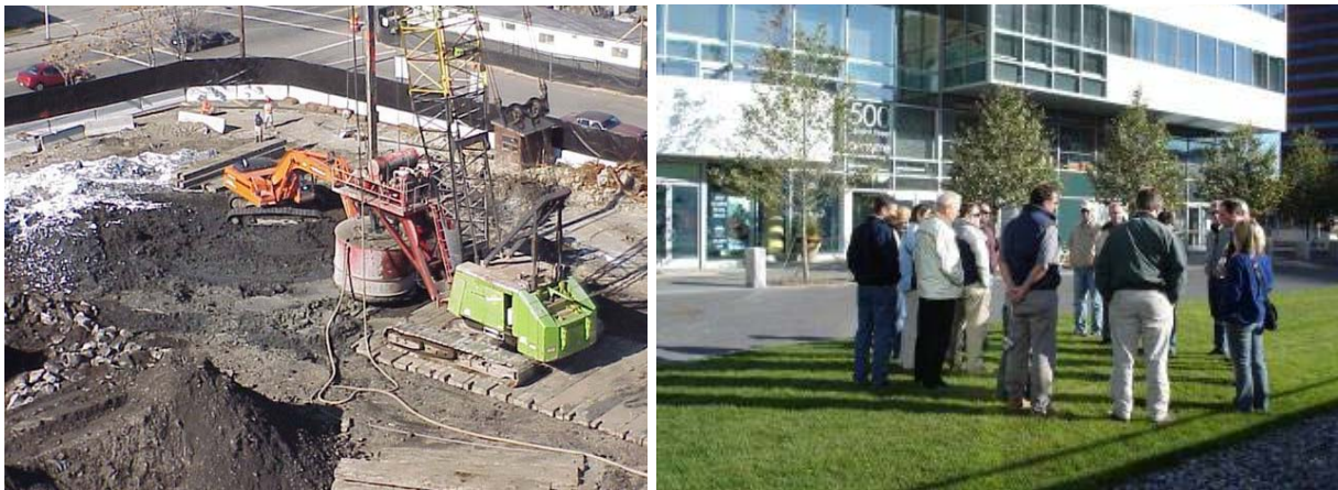
Figure 8-2. Auger-mixed in situ S/S treatment of a former MGP site in Kendall Square, Cambridge, Massachusetts (left) and after redevelopment (right). Source: Portland Cement Association; Carleo, Clark, and Wilk 2006.
