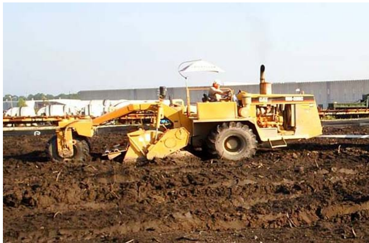
Figure A-5. S/S treatment of relocated dioxin-contaminated sediment by rotary mixer at Naval Construction Battalion Center, Gulfport, Mississippi. Source: ECC.
