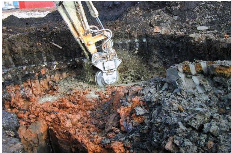
Figure A-10. S/S treatment by rotary blender at former wood-preserving site, Port Newark, N.J. Source: Key Environmental, Inc.
