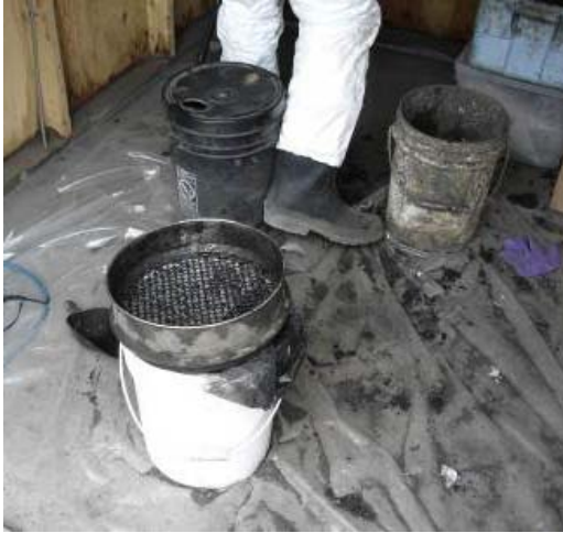
Figure 6-5. Sieve screening of treated material sample in preparation of UCS cylinder molding. Source: CETCO Contracting Services Co.
