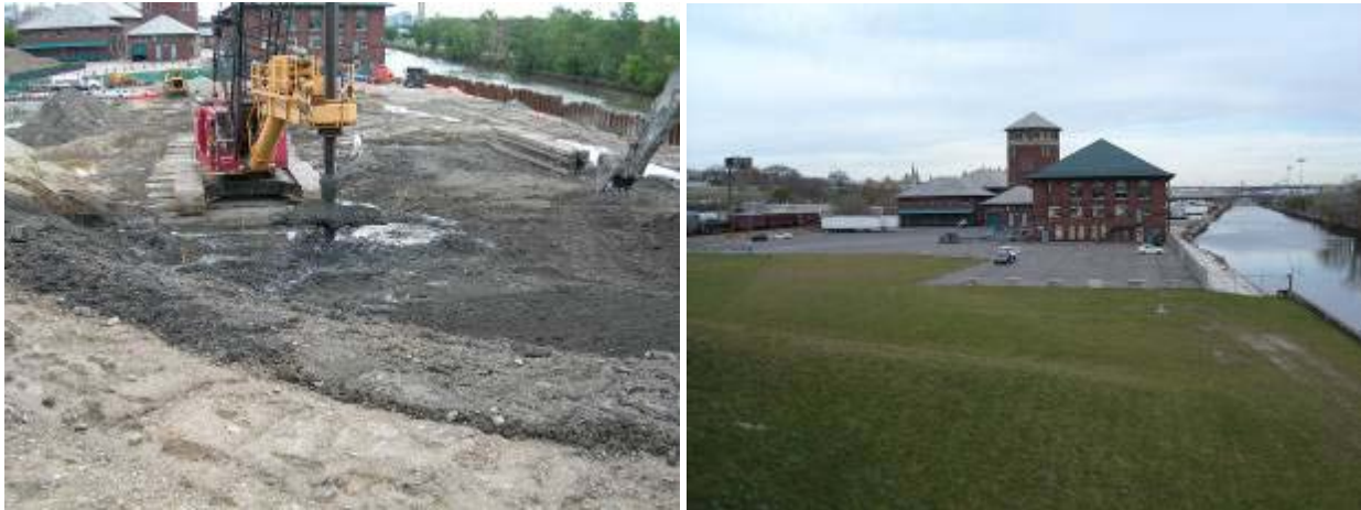
Figure 8-1. Auger-mixed in situ S/S treatment of a former MGP site in Milwaukee, Wisconsin (left) and post-treatment (right). Source: Portland Cement Association.
