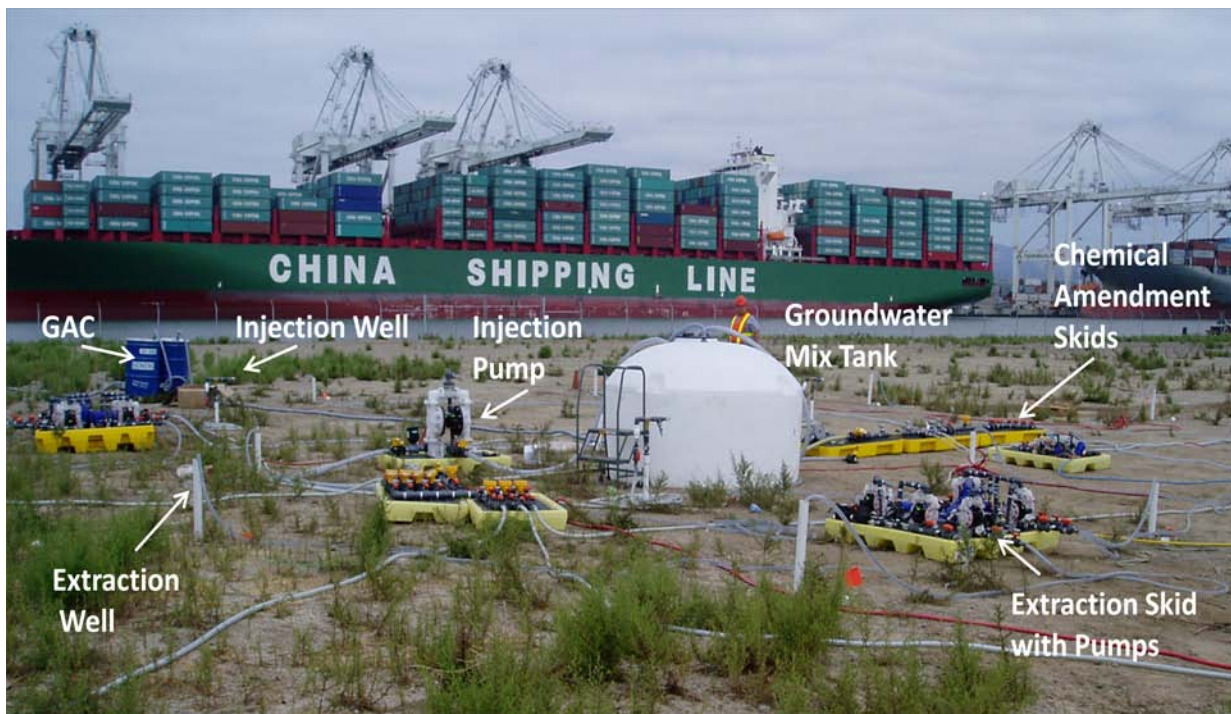
Figure 5-7. Injection and Extraction Equipment
