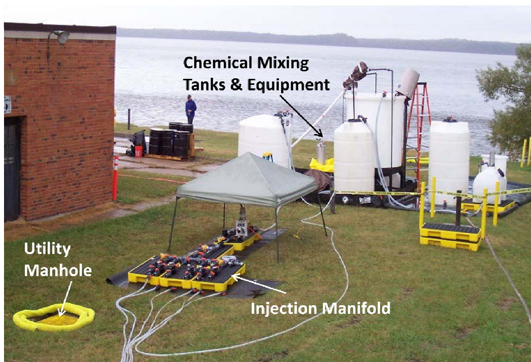
Figure 4-4. Chemical Mixing and Injection Equipment
