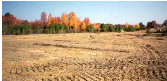
Figure 5-2. Process of developing the grade on a site and (background) example of the equipment used for grading (courtesy Charles Harman, AMEC Earth & Environmental, Inc.).
