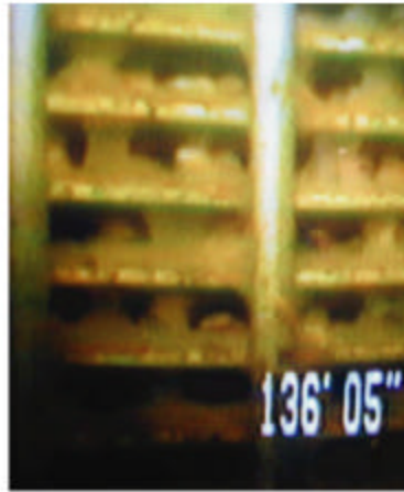
Fouled Well Screen
