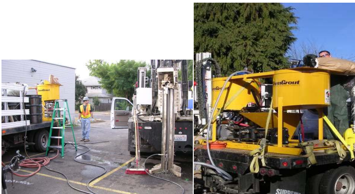
Figure 4-7. EHC mixing and injection equipment.
