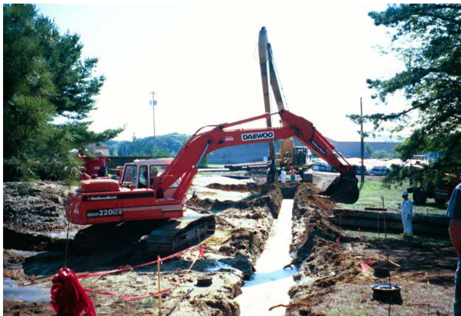
Figure 5-3. Guar slurry used during biopolymer PRB construction.
