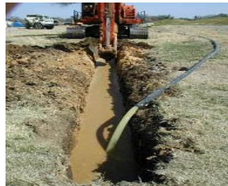
Figure 6-4. Biopolymer trench construction.
