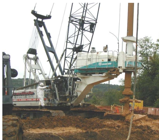
Figure 6-7. ZVI-clay application using soil mixing. (Courtesy of the U.S. Air Force)
