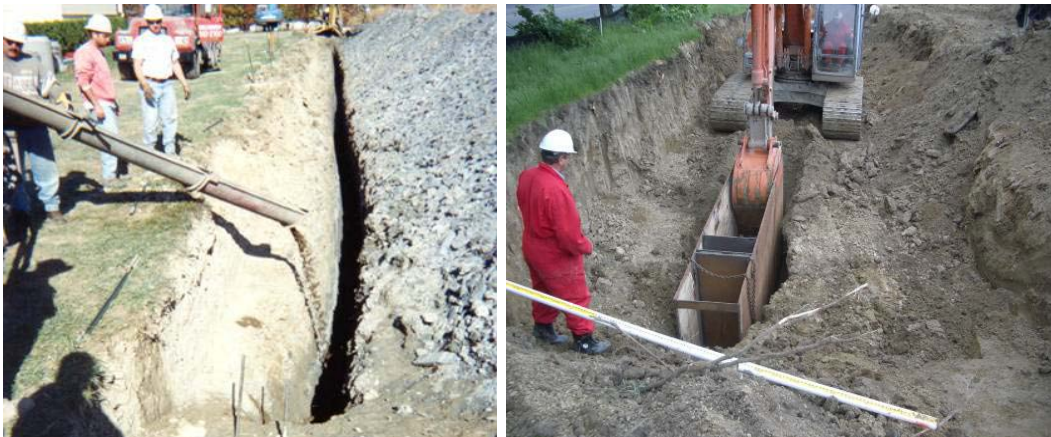
Figure 6-2. Unsupported excavation (left) and temporary trench box (right).
