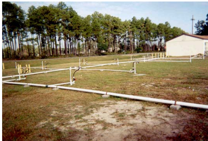
Figure B-1. MPE Extraction Wells
