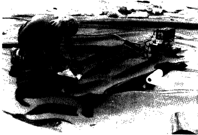
Figure 7.5(a). Two sheets of liner being cleaned and prepared for trial seaming.
