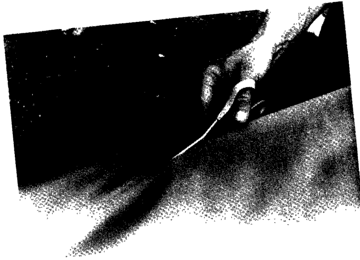
Figure 9.1(a). Trimming of excess geomembrane to obtain proper overlap prior to seaming.
