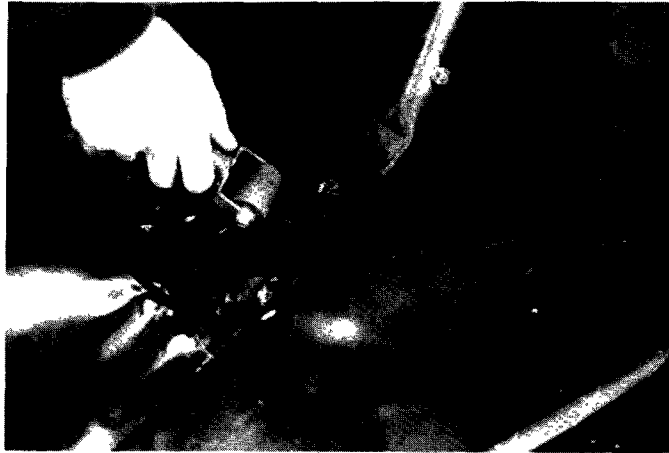
Figure 8.3(c). Overlapping and seaming the ends of the upper geomembrane to the lower geomembrane.
