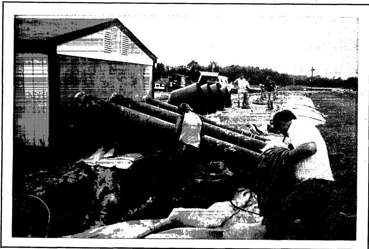
Figure 8.4 - Photograph of HDPE Smooth Wall Pipe Risers Used as Primary and Secondary Removal Systems from Sump Area to Pump and Monitoring Station.
