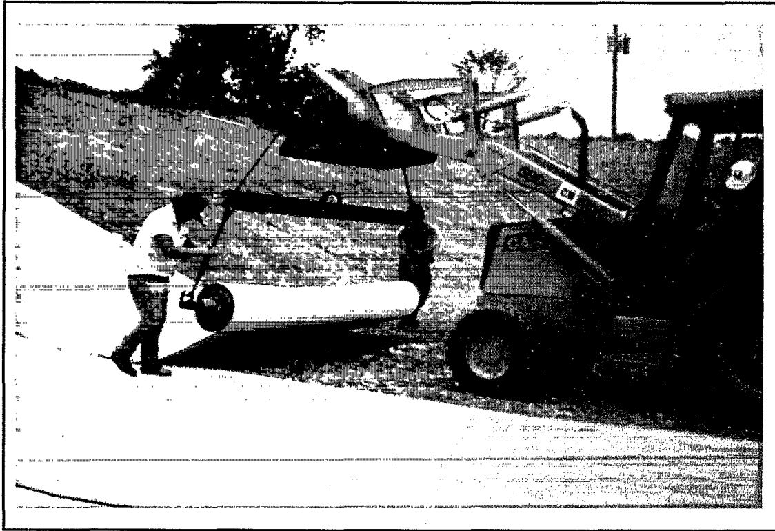
Figure 4.6(a) - Field Deployment of a GCL on a Soil Subgrade
