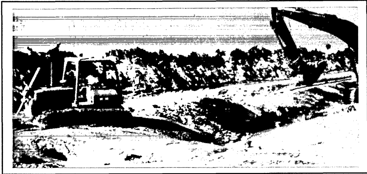
Figure 7.12 - Mixing Backfill with Bentonite Slurry.
