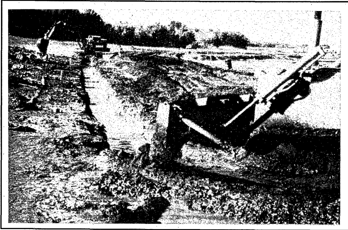
Figure 7.13 - Pushing Soil-Bentonite Backfill Into Slurry Trench with Dozer.
