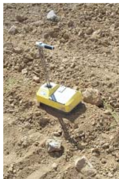
Figure 5-2. Nuclear gage determination of alternative cover layer compaction.
