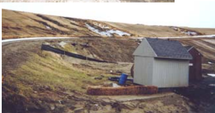
Figure 6-5. Poor cover design, resulting in both surface-water erosion failure (left) and sloughing of cover system due to excess buildup of pore water in cover drainage layer (below).
