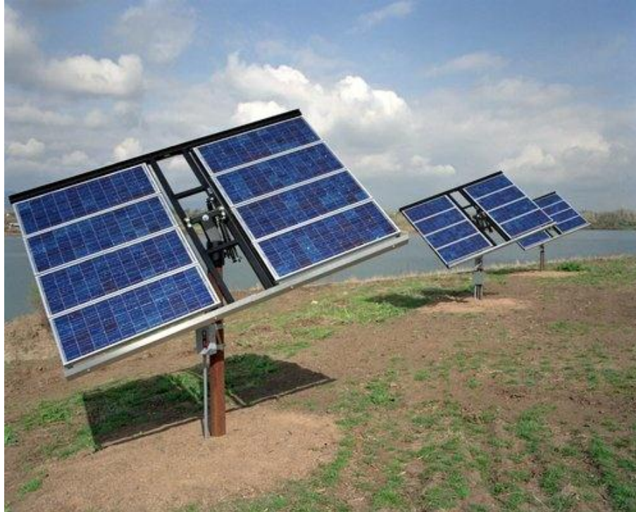
Figure 3-8: PV system with dual-axis trackers
