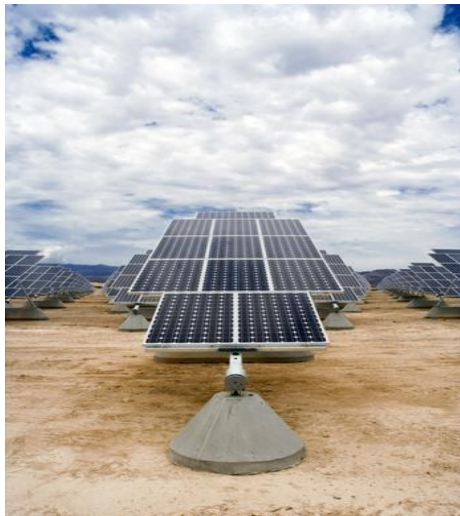
Source: NREL PIX 15280
