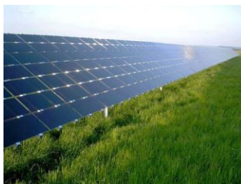
Source: NREL PIX 14726
