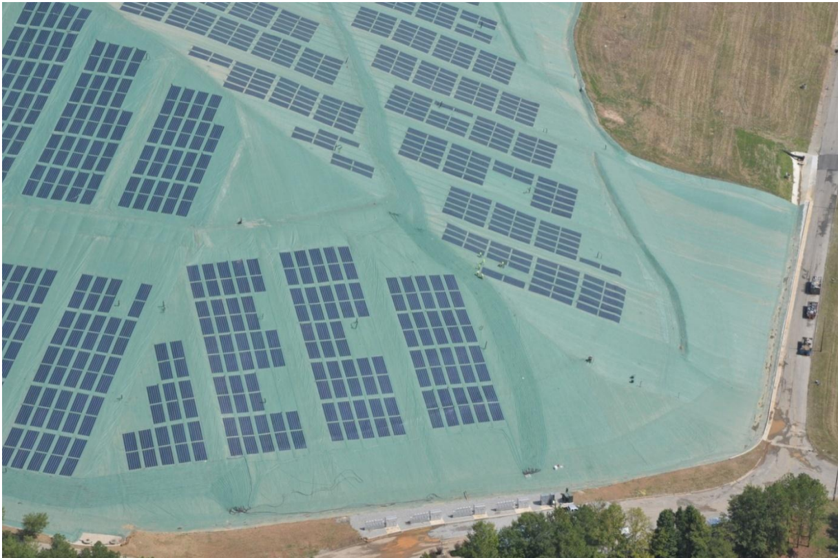
Figure 5-4: Hickory Ridge Road Landfill – Geomembrane solar cover
