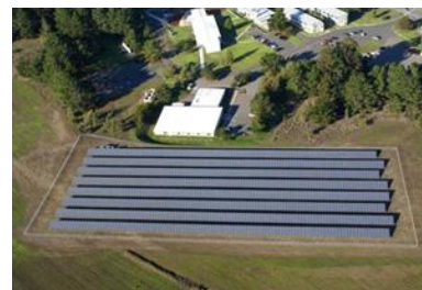
Source: NREL PIX 17395
