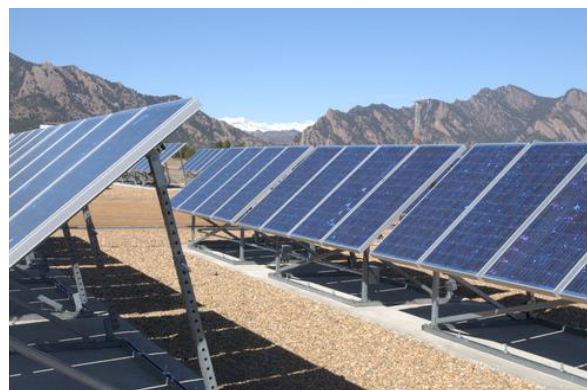
Figure 5-2: Slab foundation for PV system at Boulder, Colorado
