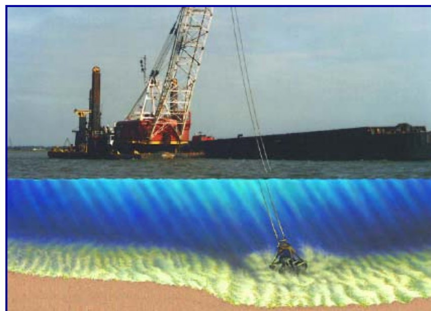
Mechanical Dredging Operation Photo courtesy of U.S. Army Corps of Engineers
