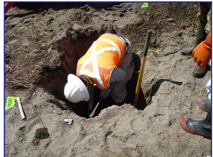
Manual MEC Removal Operations
