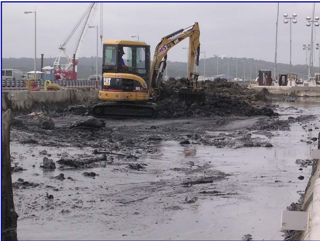
Dredge Spoils Screening Operation
