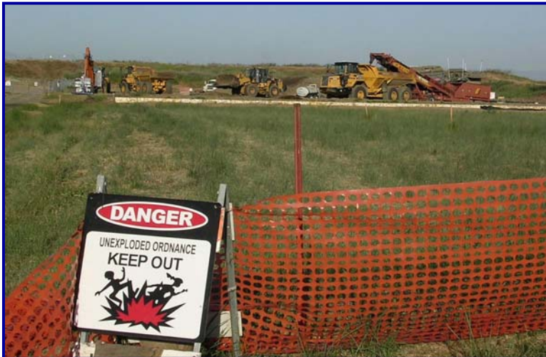
Mechanized MEC Operations
