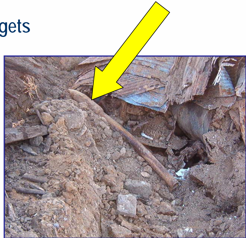
Typical Landfill Surprise
