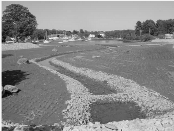
Figure 1. Salt Marsh Establishment After Consolidation and Backfilling
