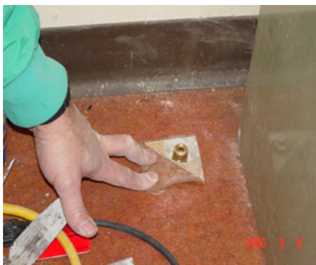
Figure G-18. Installation of subslab soil gas sample port.
