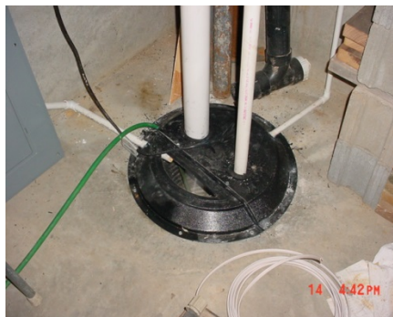
Figure J-2. Passive sump mitigation system.
