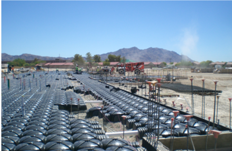
Figure J-4. Cupolex aerated floor system.
