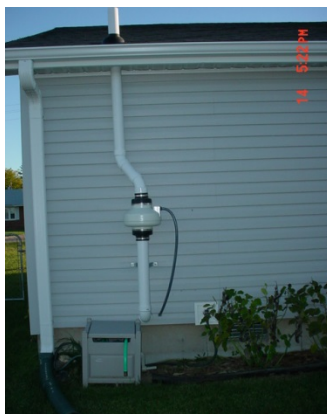
Figure J-3. Active SSD system.
