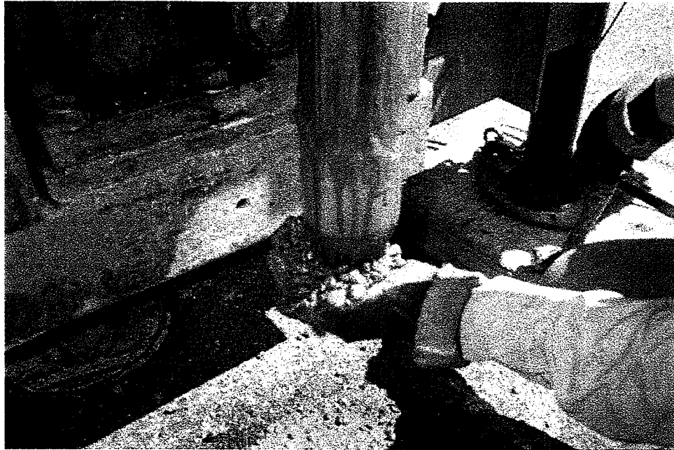
Figure 4-5. Pea Gravel Being Removed from Drive Casing
