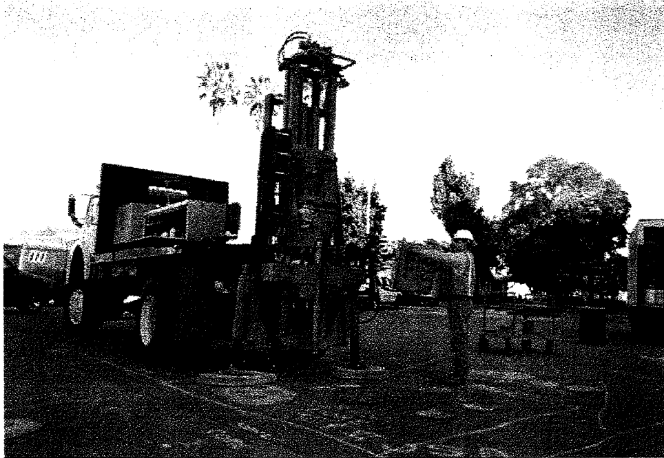
Figure 4-3. Rig Used to Collect Iron Core Samples from the Moffett Field PRB
