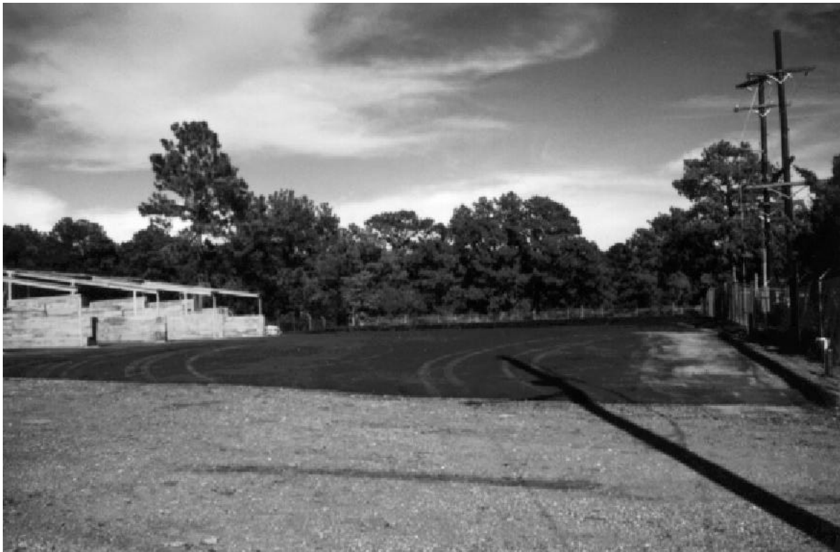
Figure 5. Asphalt pad with bermed sides built to house the vendors' plants. The pad was graded into a containment pond at the far end. Processed soil storage bins are on the left, and pole transformers are on the right.
