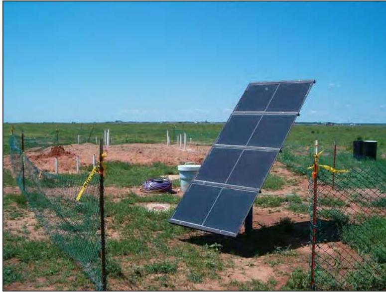
**Figure 2.1 Solar Panel to Power an Extraction Pump for the Remote Bioreactor Site at LF-03, Altus AFB, Oklahoma**
