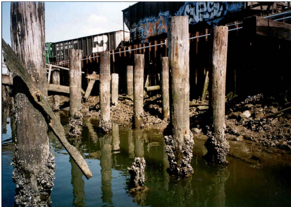
Figure 4-6. Residual Sediment Around Pilings Can Reduce the Effectiveness of Dredging
