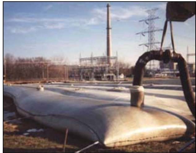
Figure 4-8. Geotextile Tube Filled with Dredged Sediment
