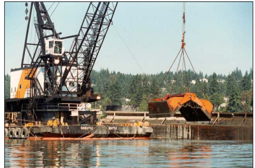
Remediating sediments at an MGP site
