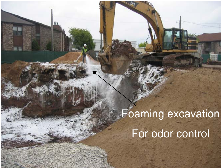
Excavating soils at an MGP site
