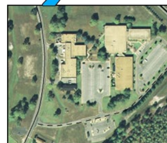
Bldg 1117 Wet Labs
